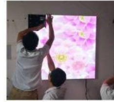
After installation Installed module
